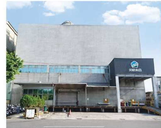
Kaohsiung Factory (Raw Material Processing)
