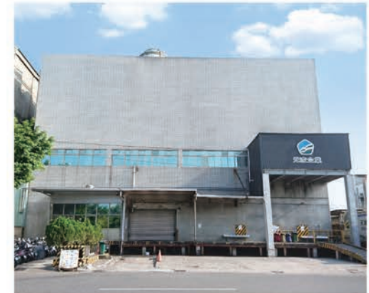
Kaohsiung Factory (Raw Material Processing)
